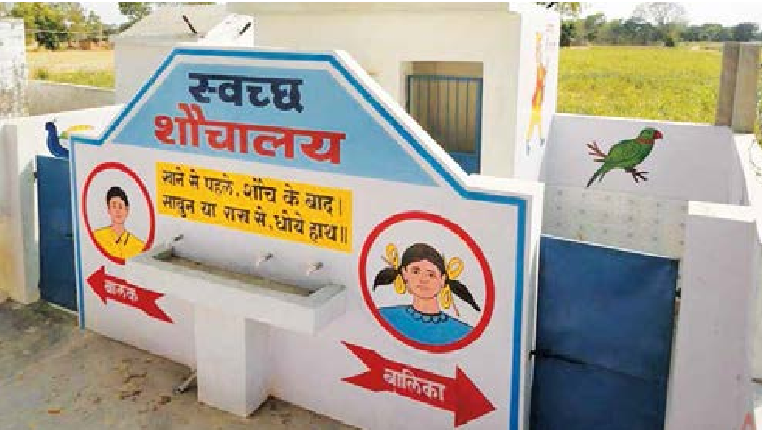
A beautifully designed toilet infrastructure built by Panchayats in Mirzapur district, Uttar Pradesh
